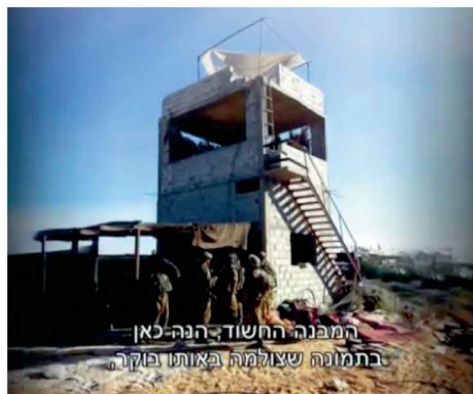
The cinder block structure above the mouth of the tunnel. The photograph is attributed to an unnamed Israeli soldier.
