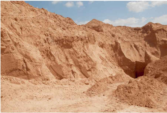
Military excavations in search of the tunnel mouth.
