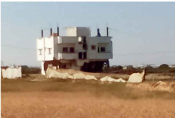
An excavation site for tunnels secured by a fence.
